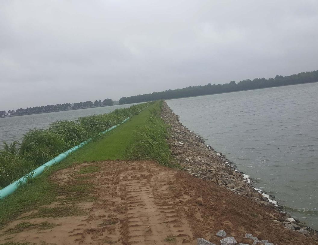
Stone pulled up onto the slope before new stone is added.
